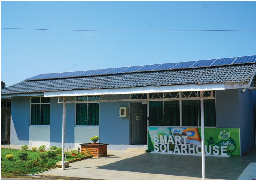
Figure 1: Exterior View of the Smart Solar House.
