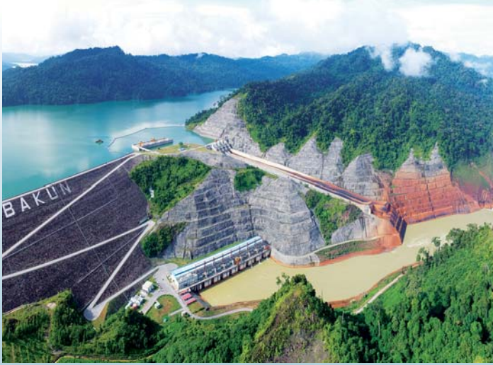
Bakun hydroelectric plant
