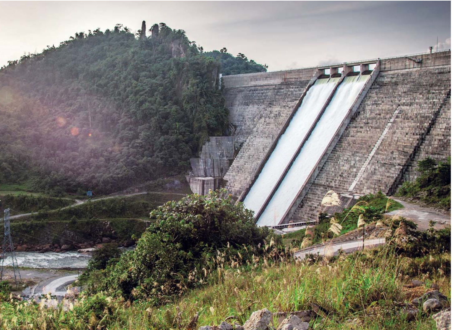
Murum hydroelectric plant
