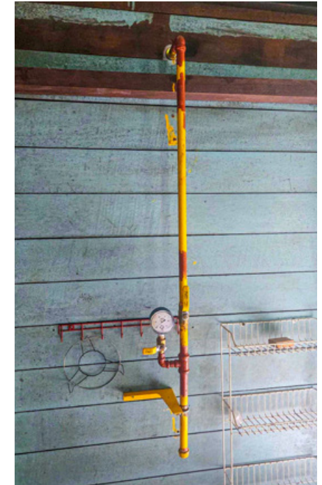
Figure 4: Internal gas pipeline installed at residents' houses in Kampung Teh and Kampung Tabo, Mukah.
