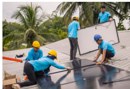
Figure 8: Installation of Solar Panels.
